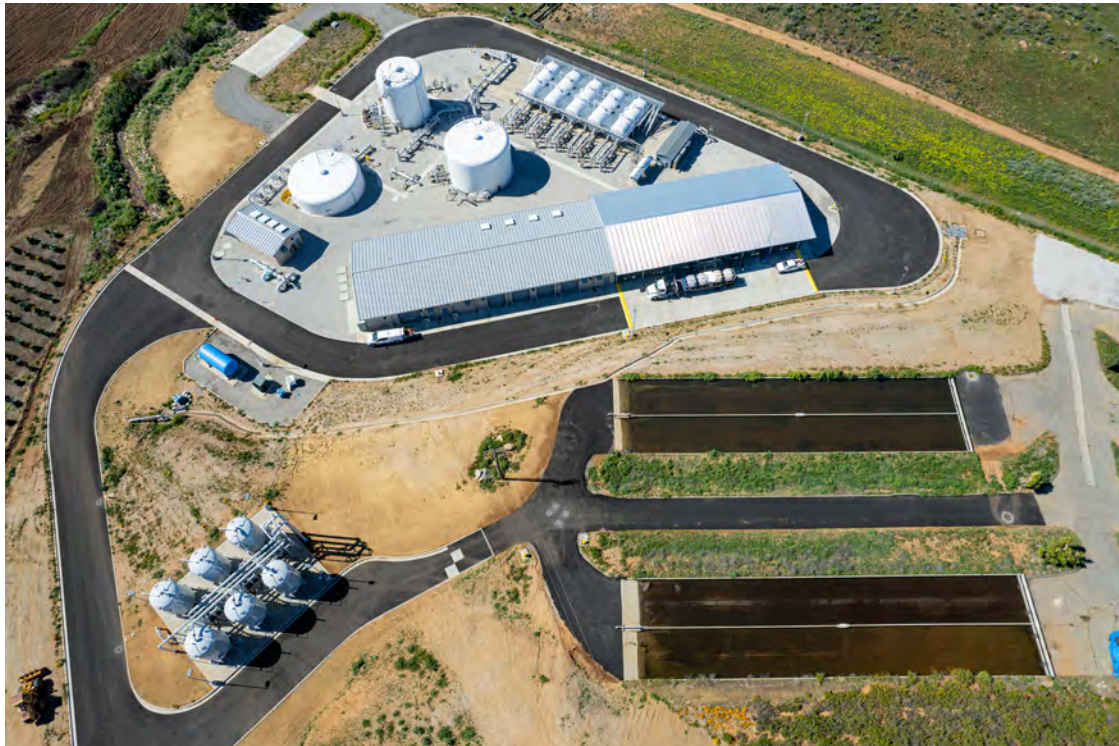
Santa Margarita Groundwater Treatment Plant
