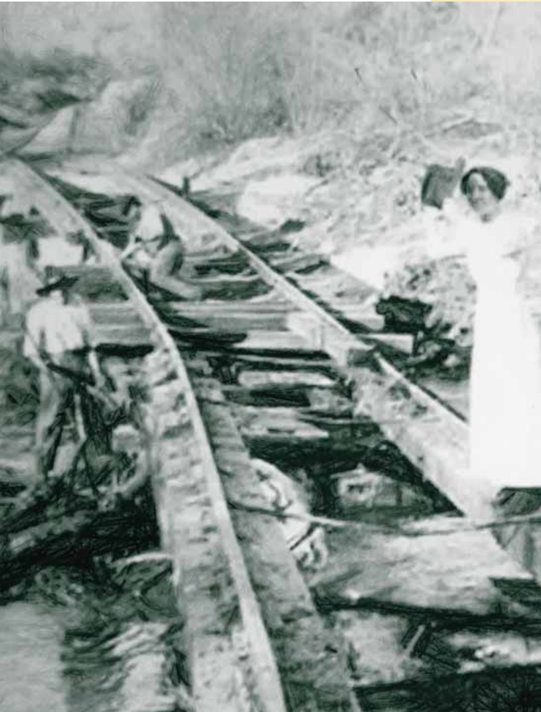
Above: Train tracks leading to and from Fallbrook suffered tremendous damage as a result of the 1916 flood along the Santa Margarita River. Courtesy of the Fallbrook Historical Society
