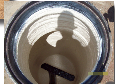
Pipeline relining program
