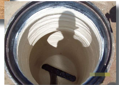
Pipeline relining program
