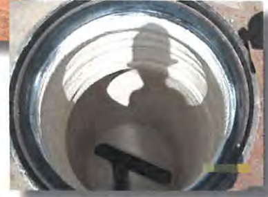
Pipeline relining program
