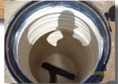
Pipeline relining program
