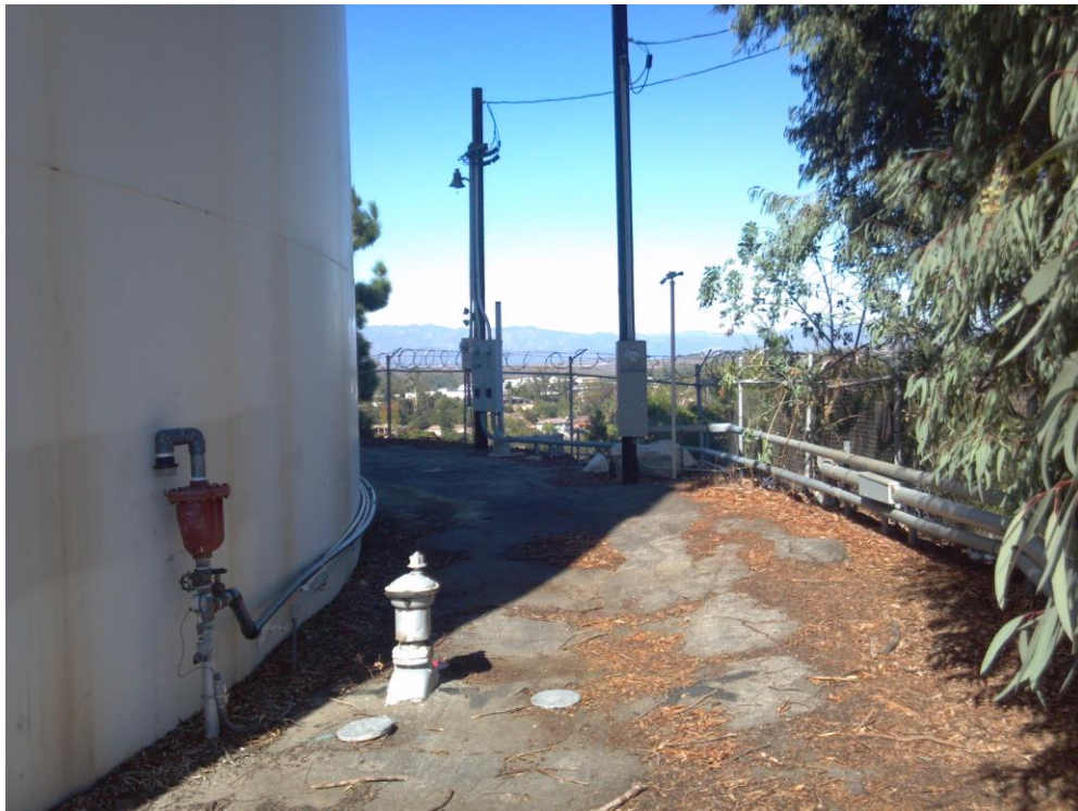
Photo No. 2: Asphalt paved pathway surrounding the Reservoir and fenced perimeter
