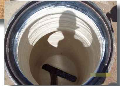
Pipeline relining program
