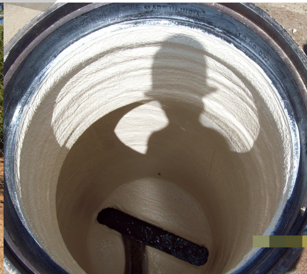
Pipeline relining program
