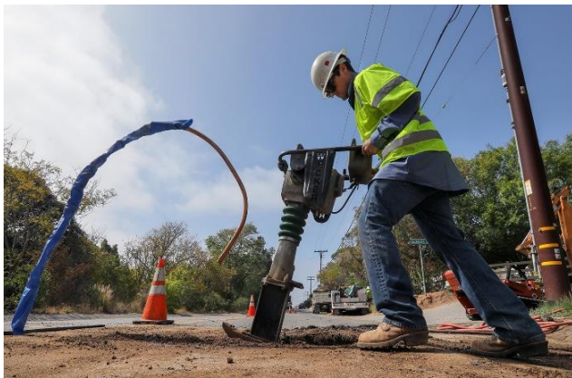
FPUD is working to rehabilitate and replace old pipelines and other aging facilities.
