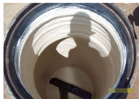
Pipeline relining program
