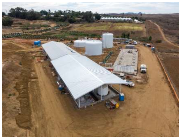
Construction progress of the SMGTP
