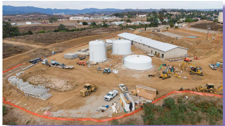
Construction progress of the SMGTP
