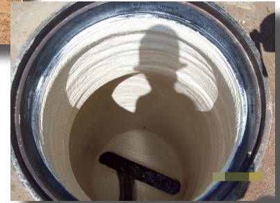
Pipeline relining program
