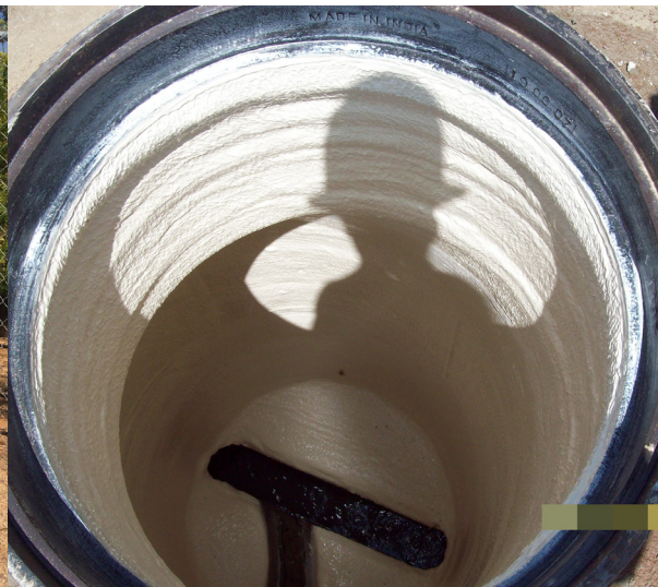
Pipeline relining program
