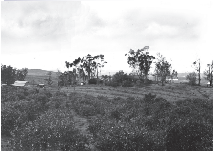
Water Reclamation Plant Alturas Road 1922
