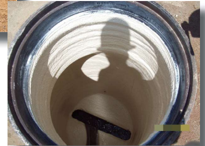
Pipeline relining program
