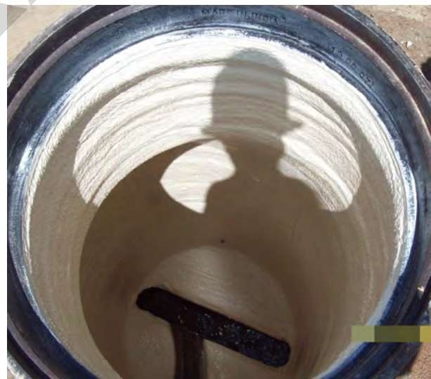
Pipeline relining program
