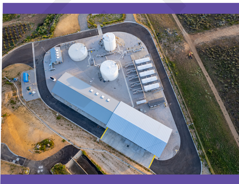
Aerial View of the SMGTP
