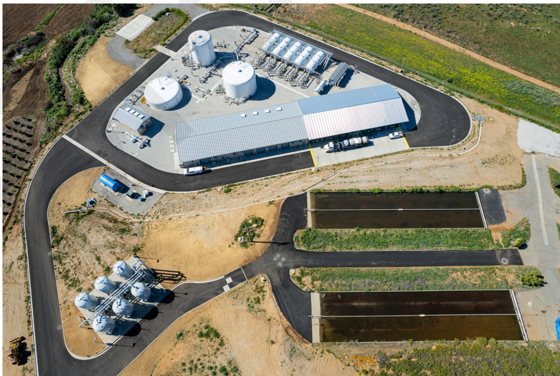
Santa Margarita Groundwater Treatment Plant
