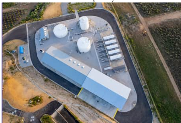
Aerial View of the SMGTP
