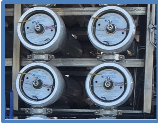
Figure 5-8 Vessel Feed/Concentrate Connections
