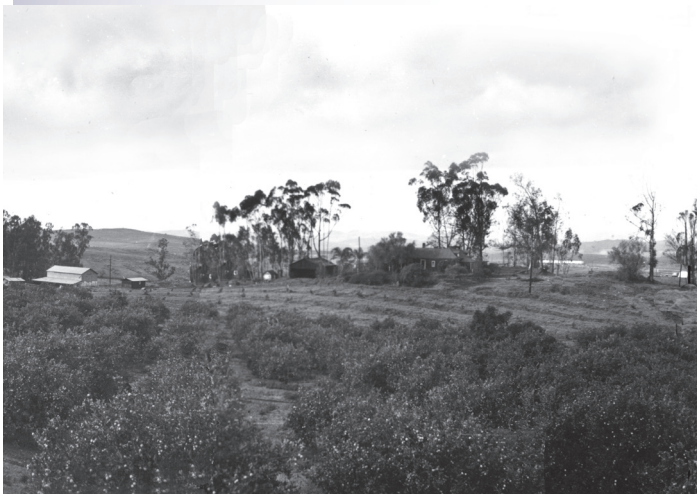
Water Reclamation Plant Alturas Road 1922
