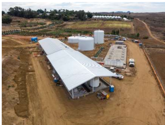
Construction progress of the Fallbrook Groundwater Treatment Plant
