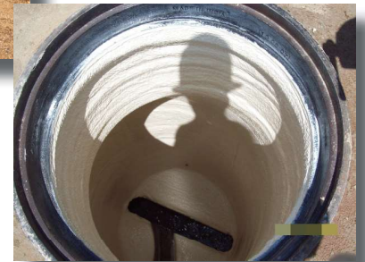
Pipeline relining program
